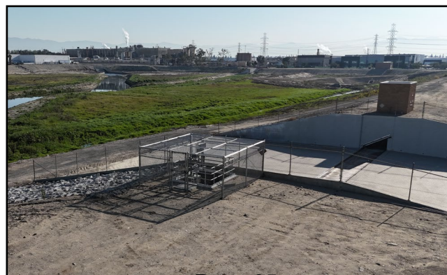
Outlet Control Gate/Rubber Dam System
